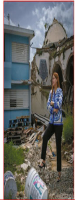
Principal Carmen Echevarria in front of the wrecked shell of Immaculada Concepcion School and Parish which was destroyed by a 6.4 magnitude earthquake.
